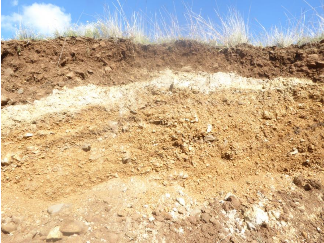
Plate 17: Alternative Site 3 Dam - Close up view of the fill profile in the above cutting.
