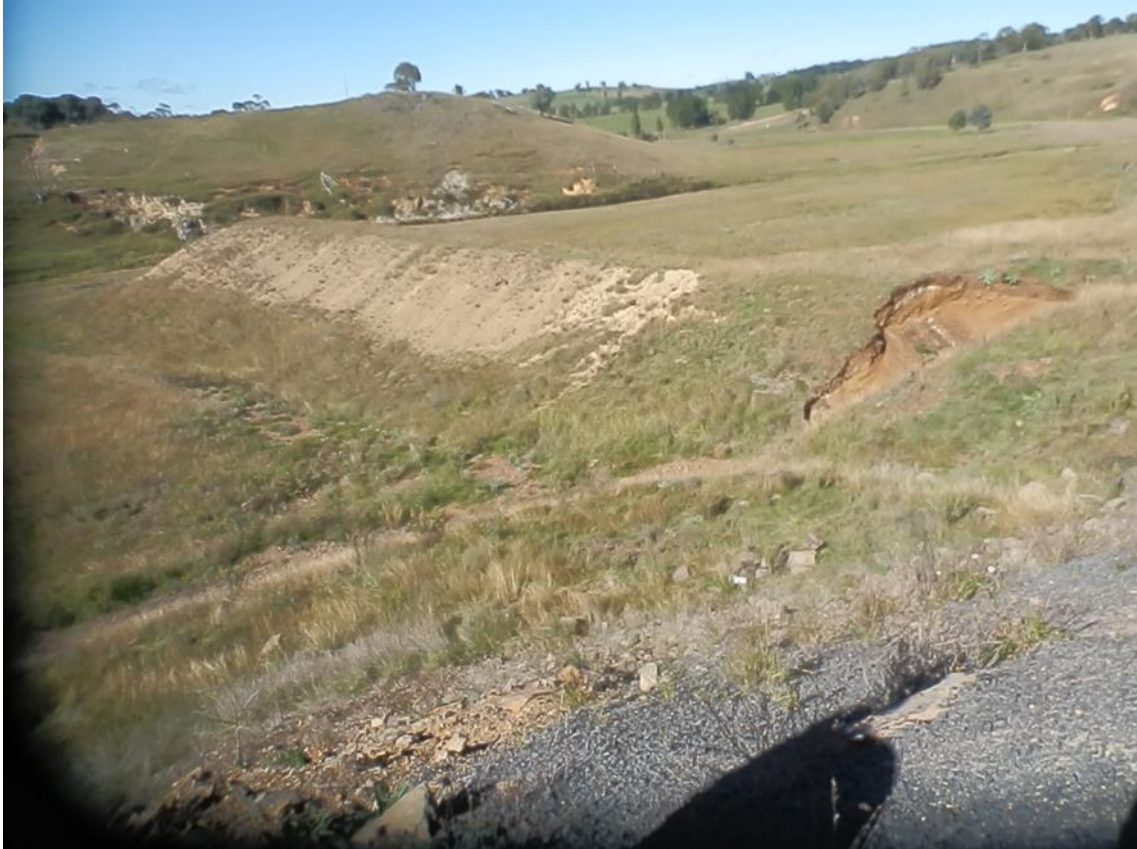
Plate 15: Alternative Site 3 Dam - General view of existing right embankment.
