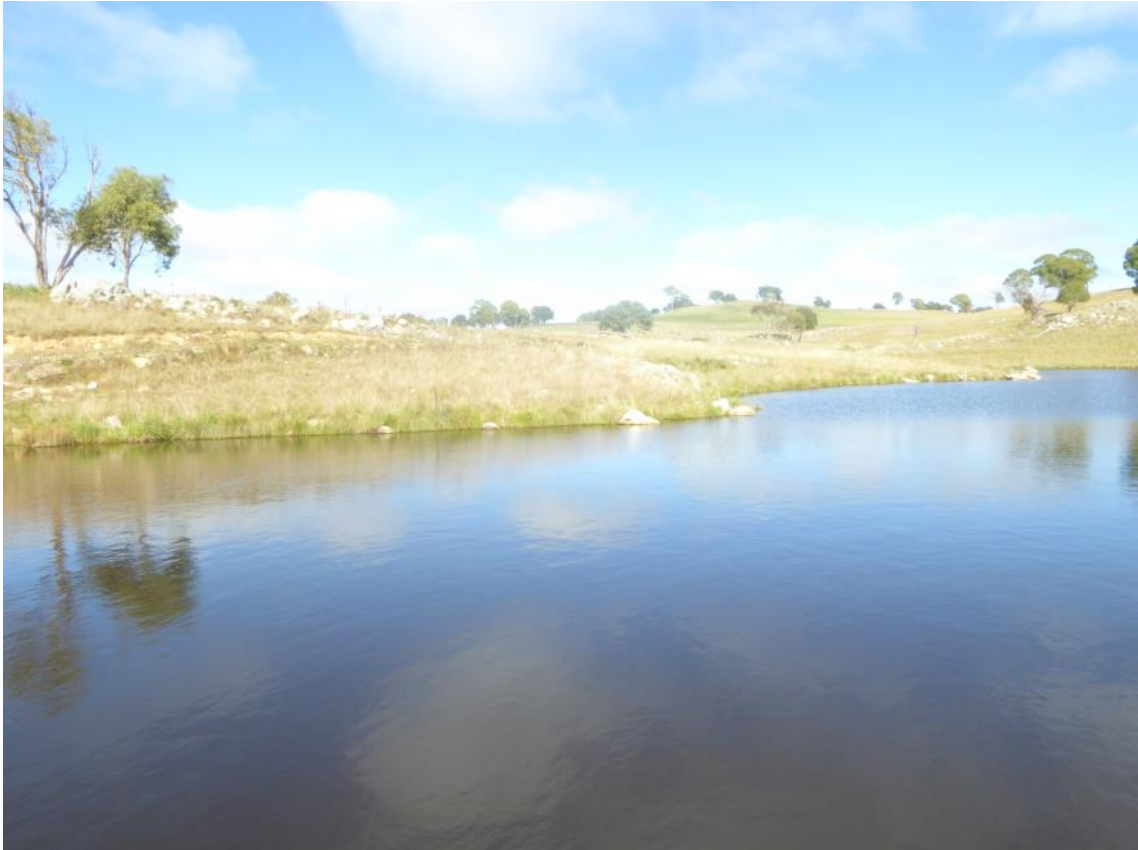
Plate 7: Guyra Dam 2 - Upstream view of the right river bank.
