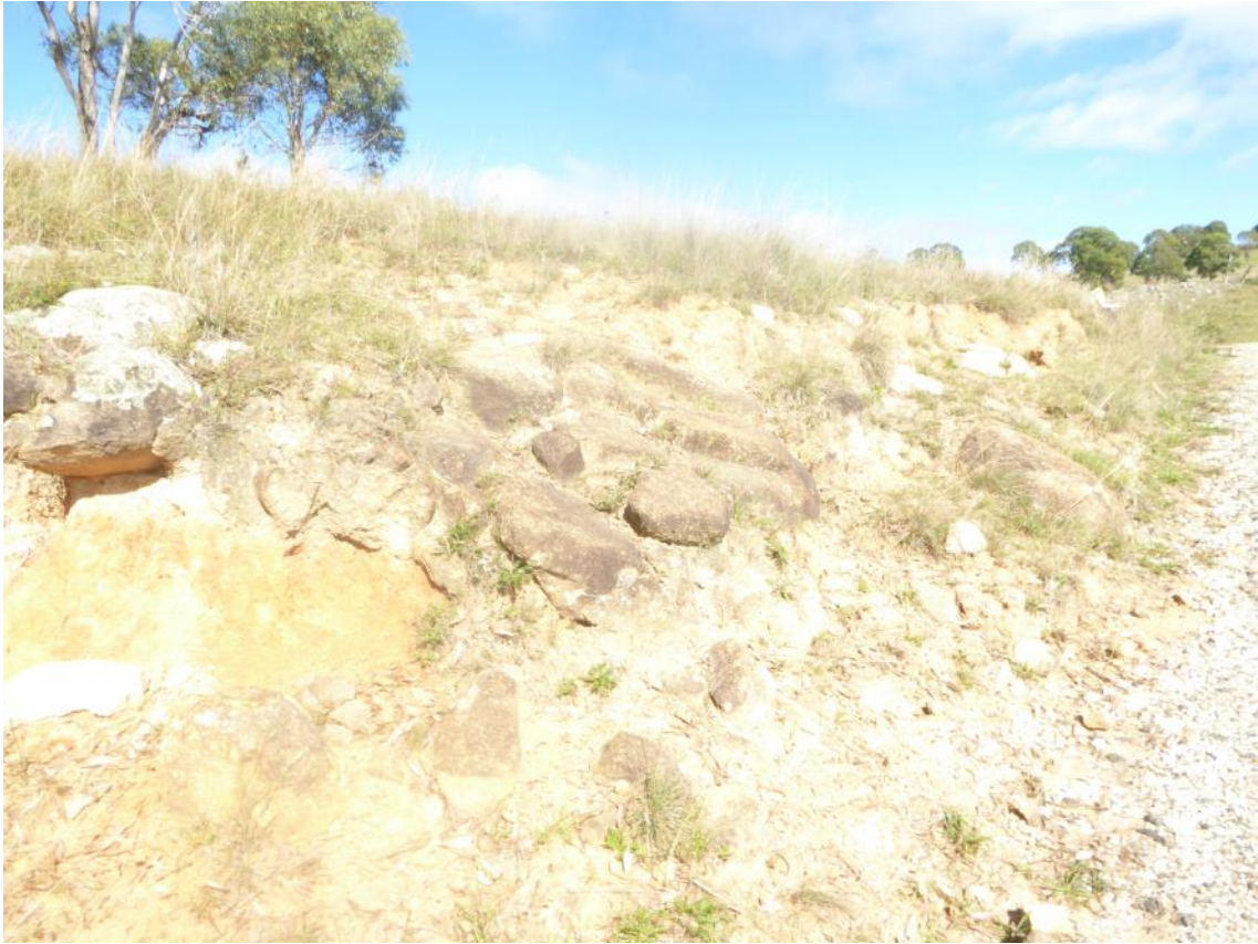
Plate 23: View of the cutting on the right bank at Guyra Dam 2, showing shallow residual boulder basalt profile overlying more deeply weathered bedrock.
