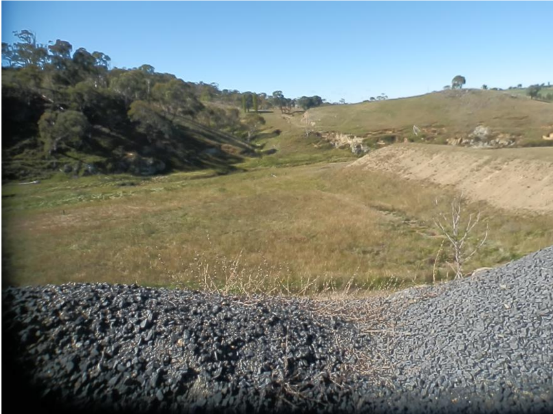
Plate 13: Alternative Site 3 Dam - General view of the site and left abutment looking south-east from the quarry.
