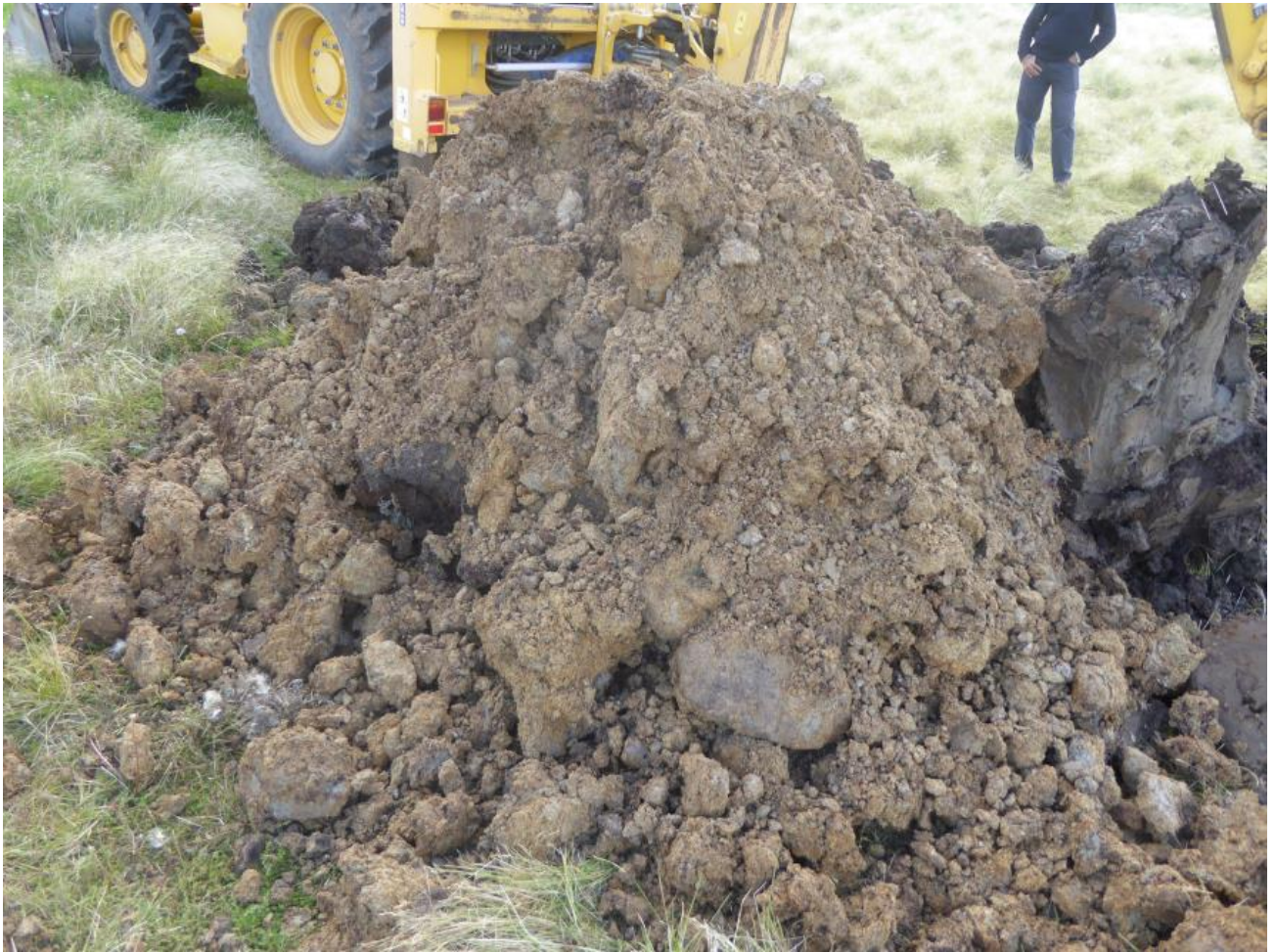
Test Pit TP1 - Stockpile.
