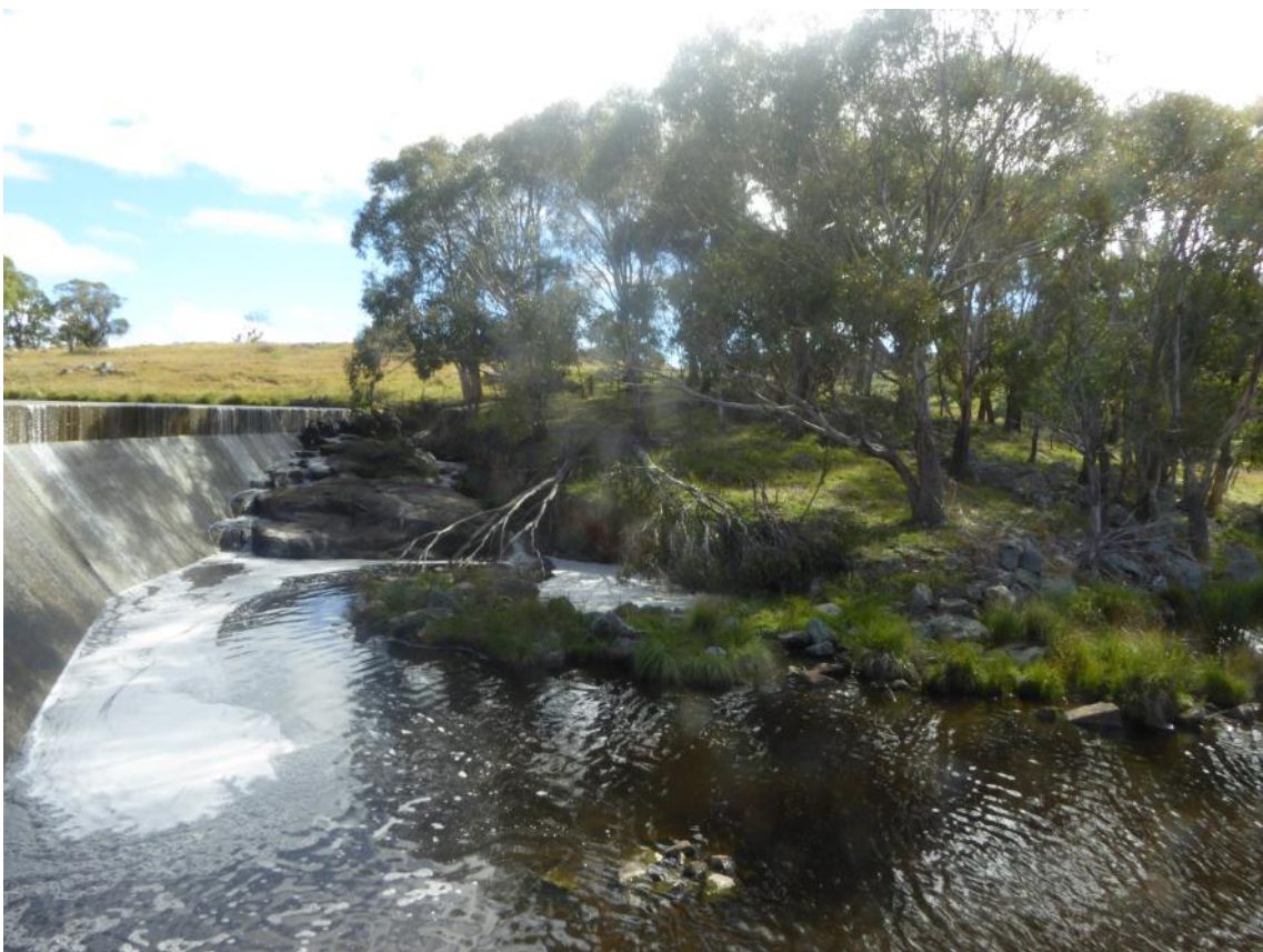
Plate 2: Guyra Dam 2 - View of the left abutment.
