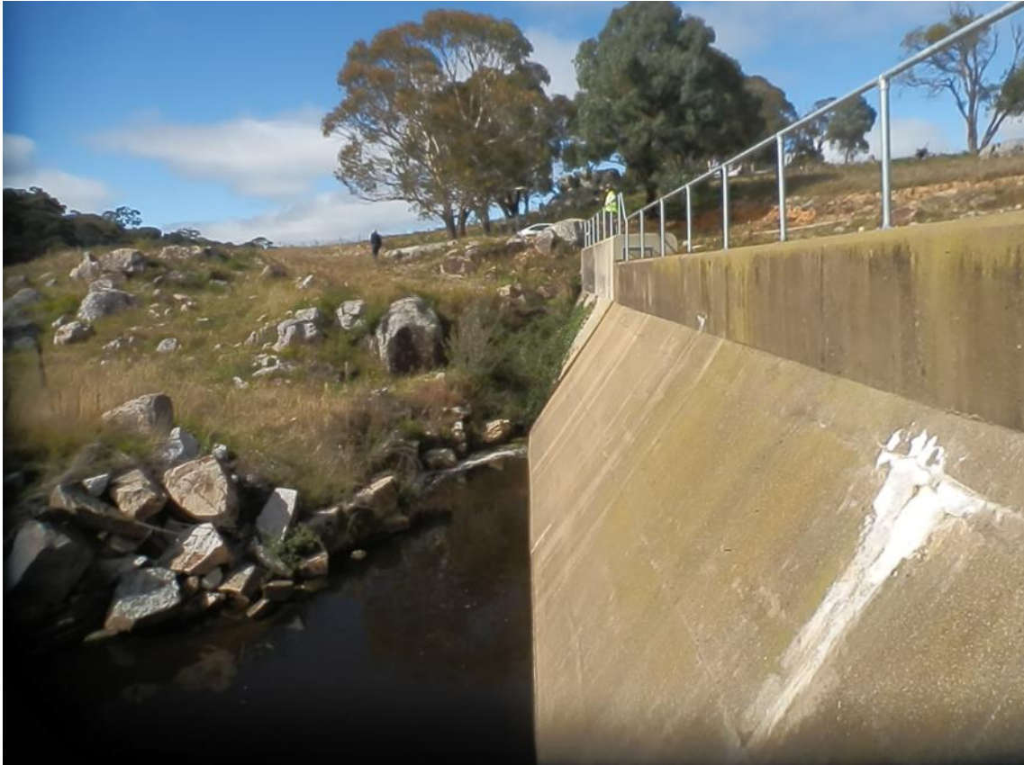
Plate 3: Guyra Dam 2 - General view of the right abutment.
