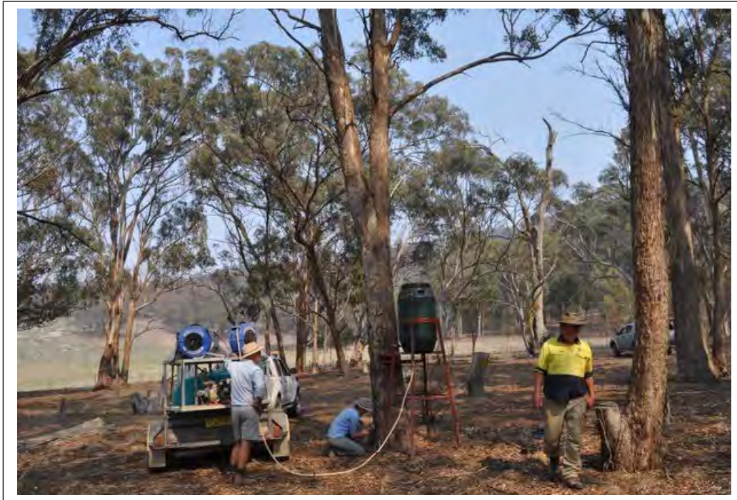
Photo 12. Koala drinker being installed by Southern New England Landcare volunteers, photo K Watson.
