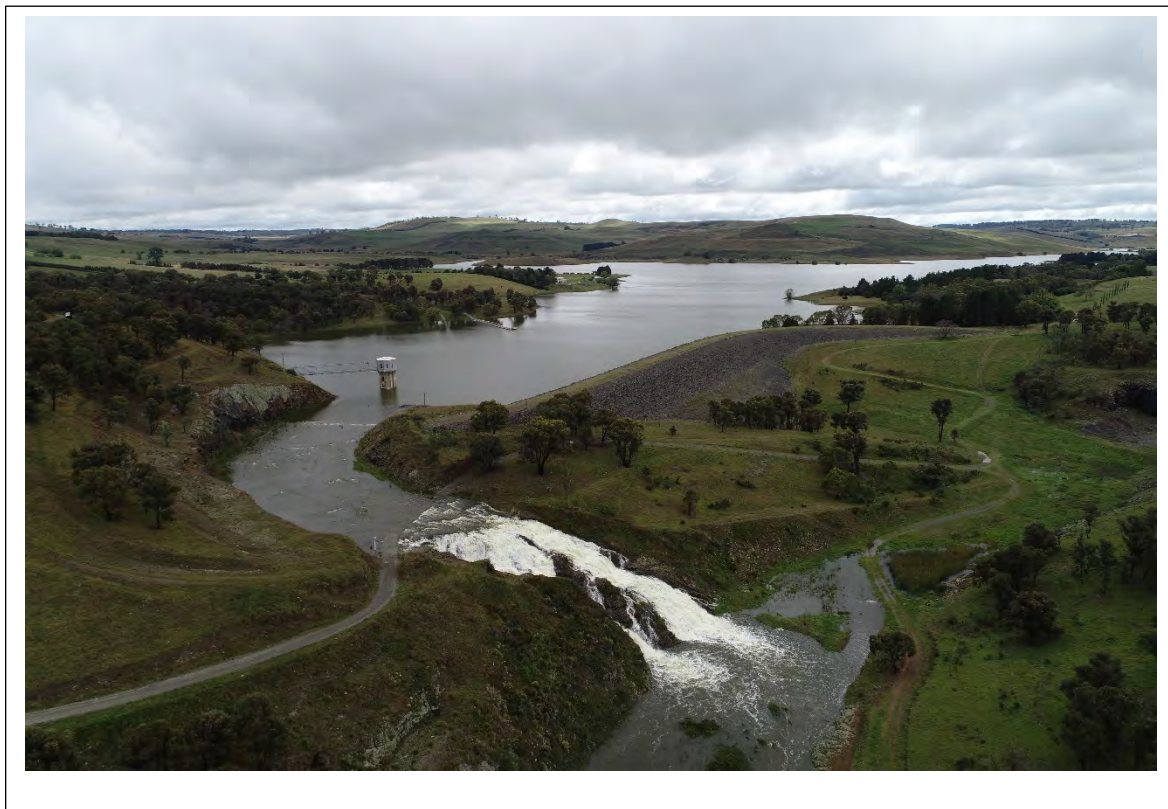
Photo 7. Malpas Dam wall overflowing on 24 th March 2021.
