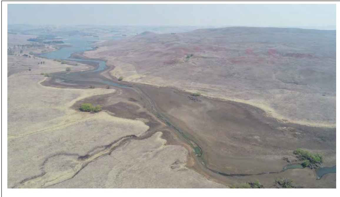
Photo 6. Malpas Dam on 24 th June 2019 looking towards the dam wall in the distance.
