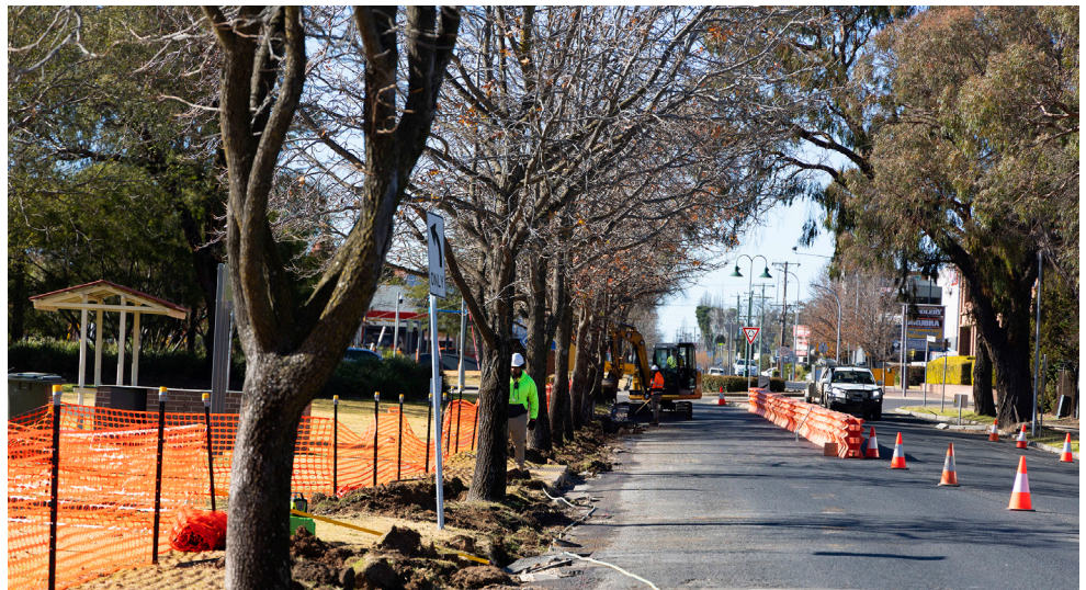
Dumaresq Street kerb and guttering
