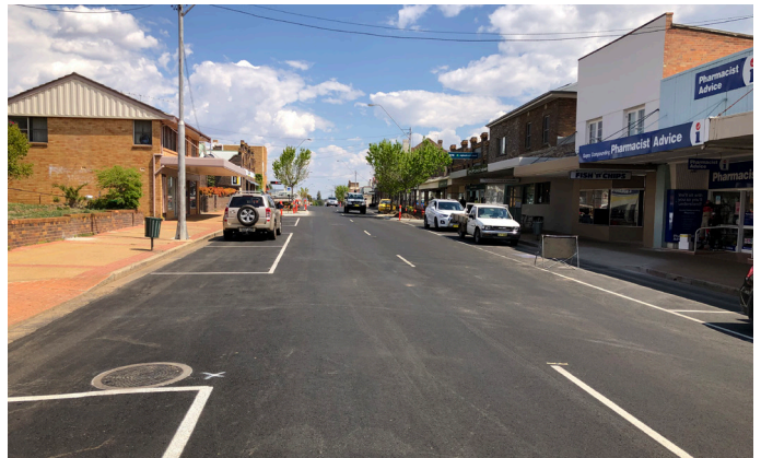
Final pavement completed
