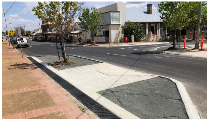
Street scaping ready for planting
