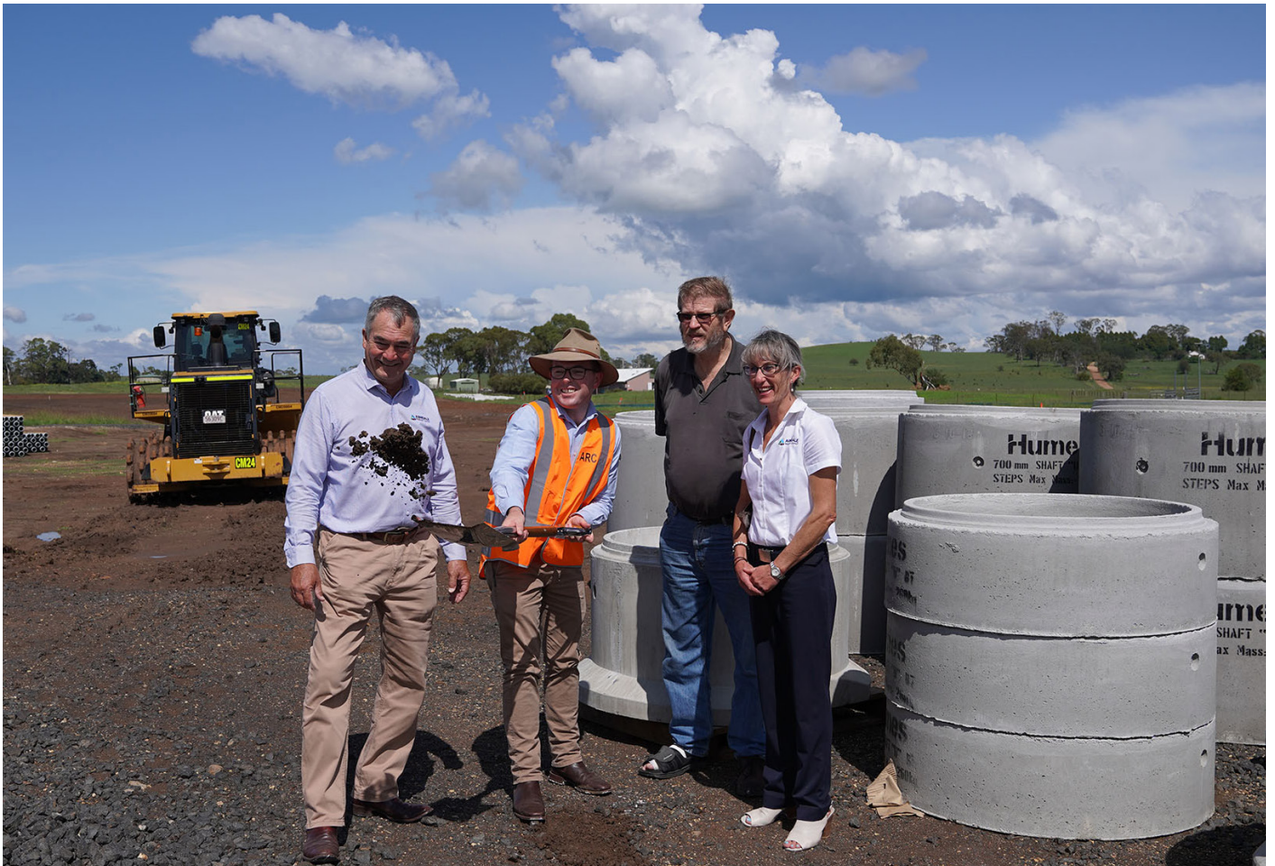
Official sod turn marking the commencement of construction works on the new business park
