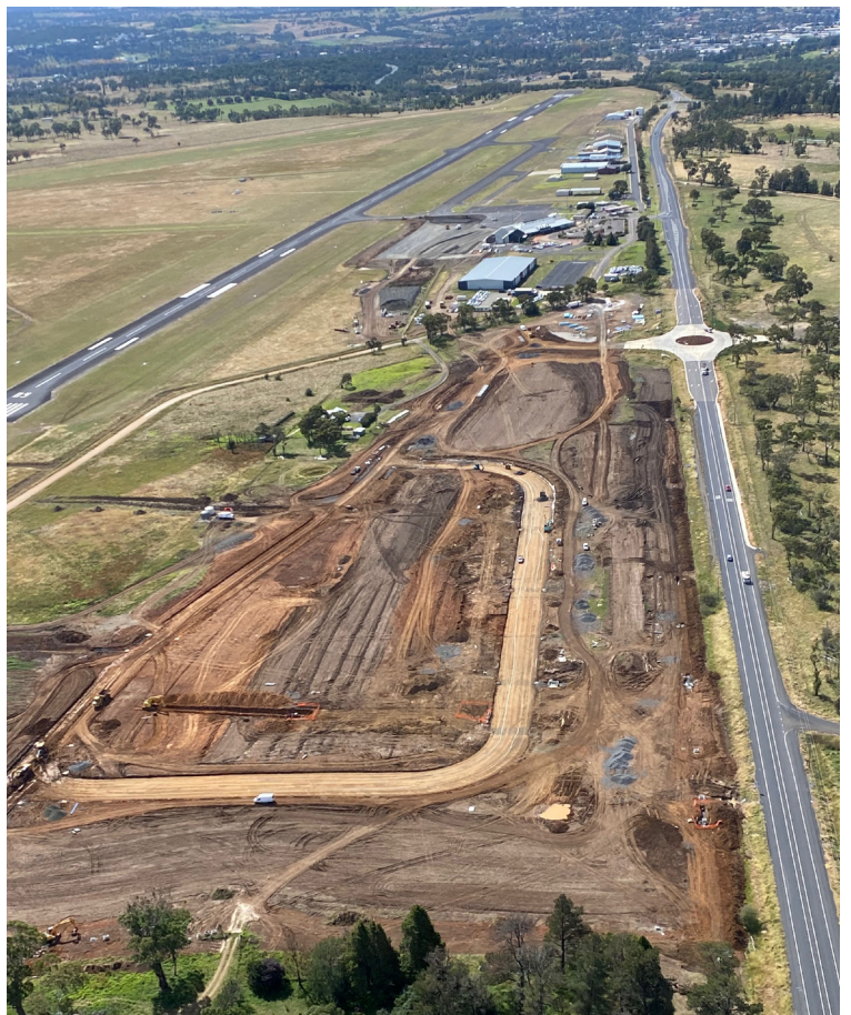
Construction on the new business park
