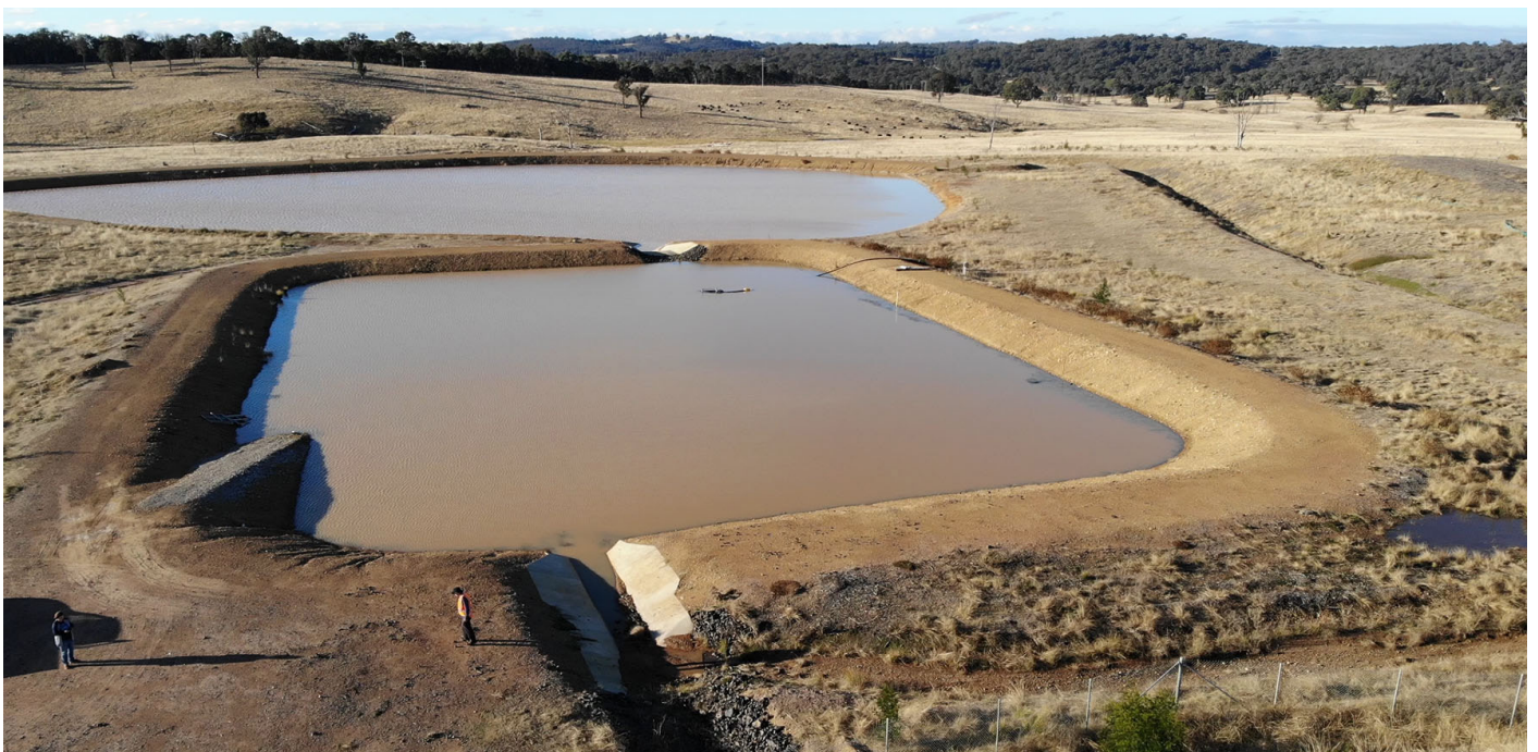
Rainfall within the landfill site but outside of an active landfill cell, contaminated by debris and sediments, is classified as 'dirty' water and is channeled into a sedimentation basin, situated downstream.
