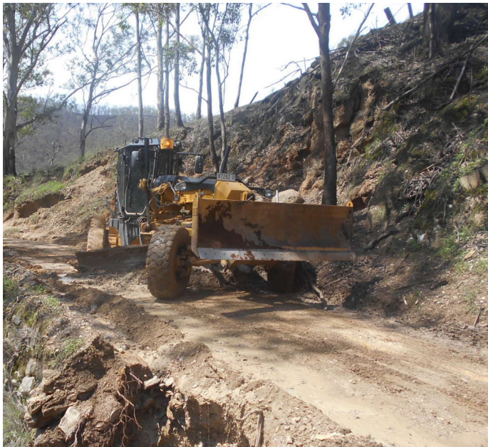
Emergency remediation works on Kempsey Road
