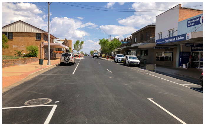
Final pavement completed
