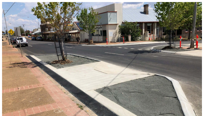
Street scaping ready for planting
