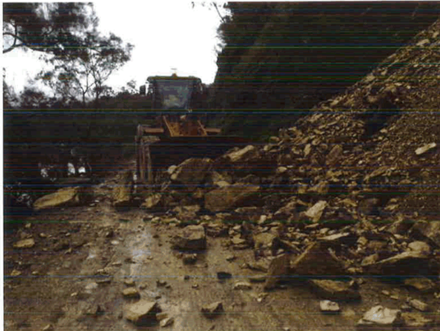
Figure 7-1 Landslip clearing works; Source ARC
