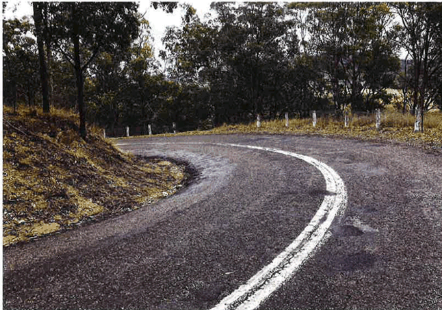
Figure 9-2 Limited sight distance on corners creates risk of control loss and side collisions
