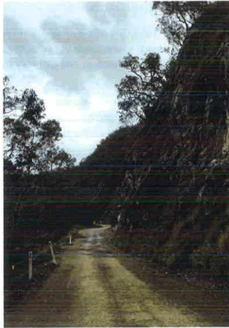
Figure 5-1 Narrow road with unsecured landslip pose risks for road users
