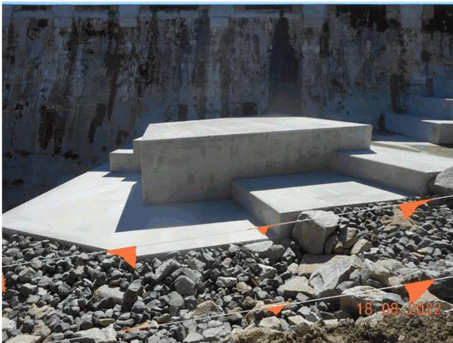
Photo Showing Encapsulated Boulder and Stepped Sections
