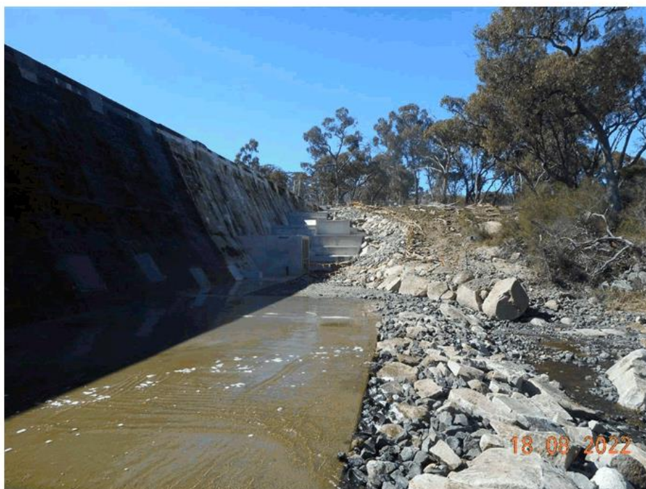
Photo Showing Completed Erosion Control Slab System and Drain
