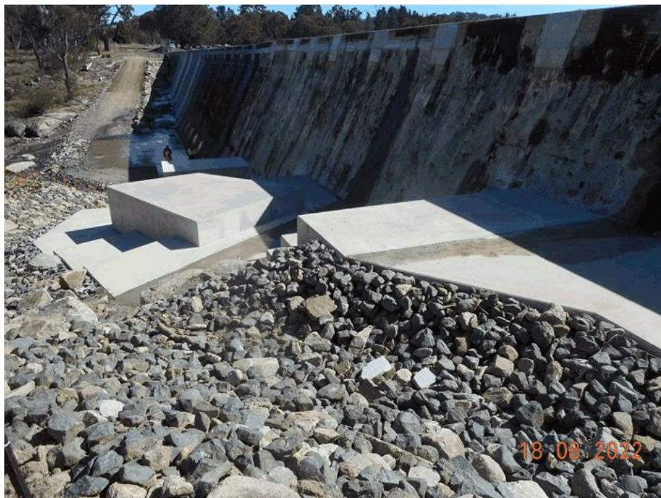
Photo Showing Closeup of Slabs above the Boulder Section
