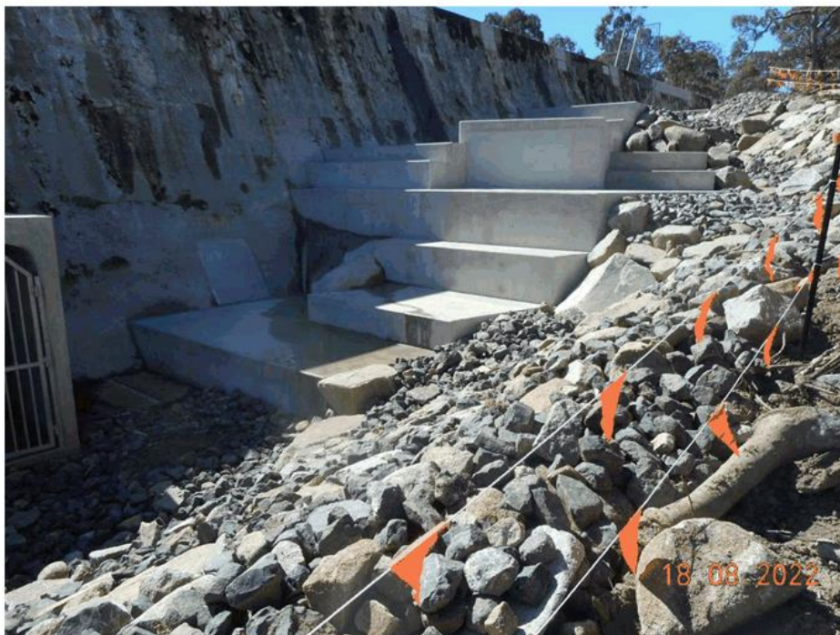
Photo Showing Encapsulated Boulder and Stepped Section
