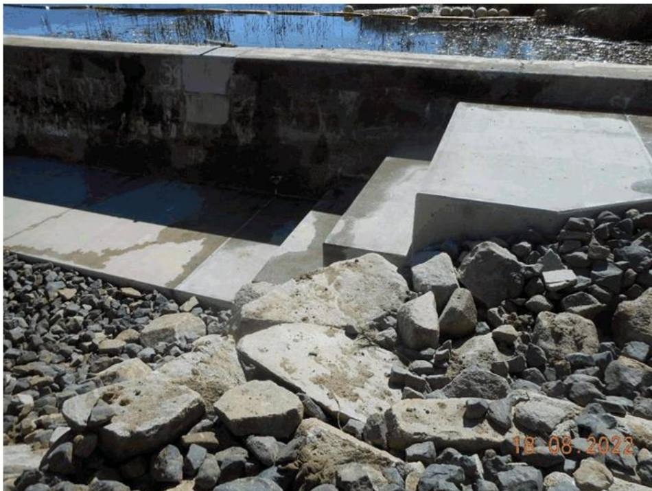
Photo Showing Upper Erosion Control "Steps" and Riprap
