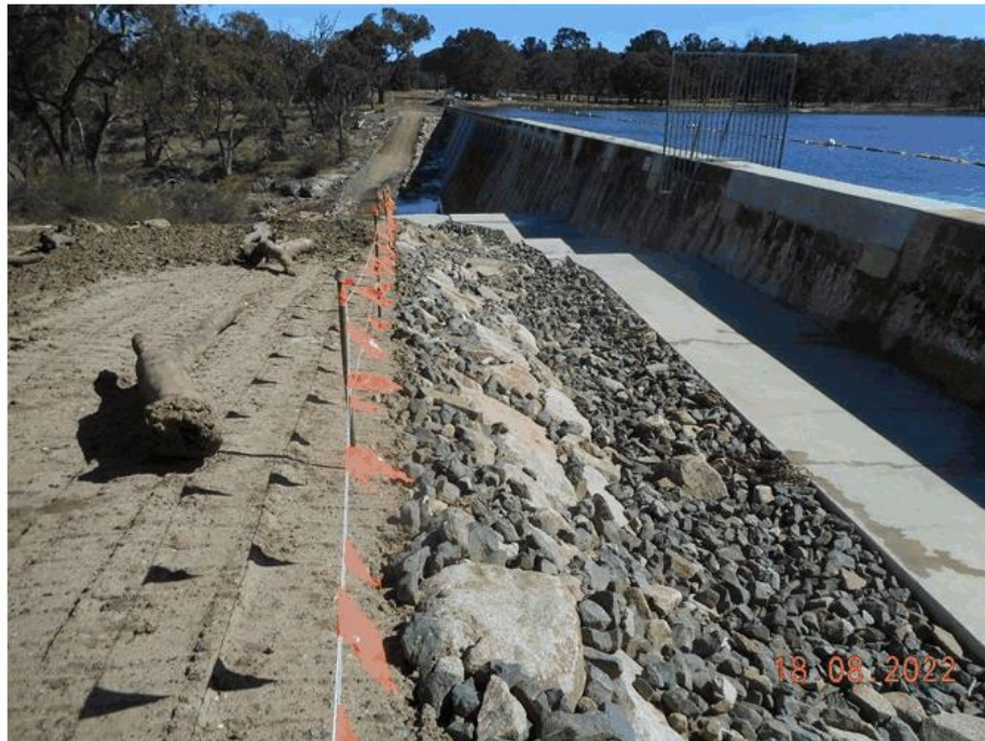
Photo Showing Completed Upper Slabs and the V Drain Riprap Placement
