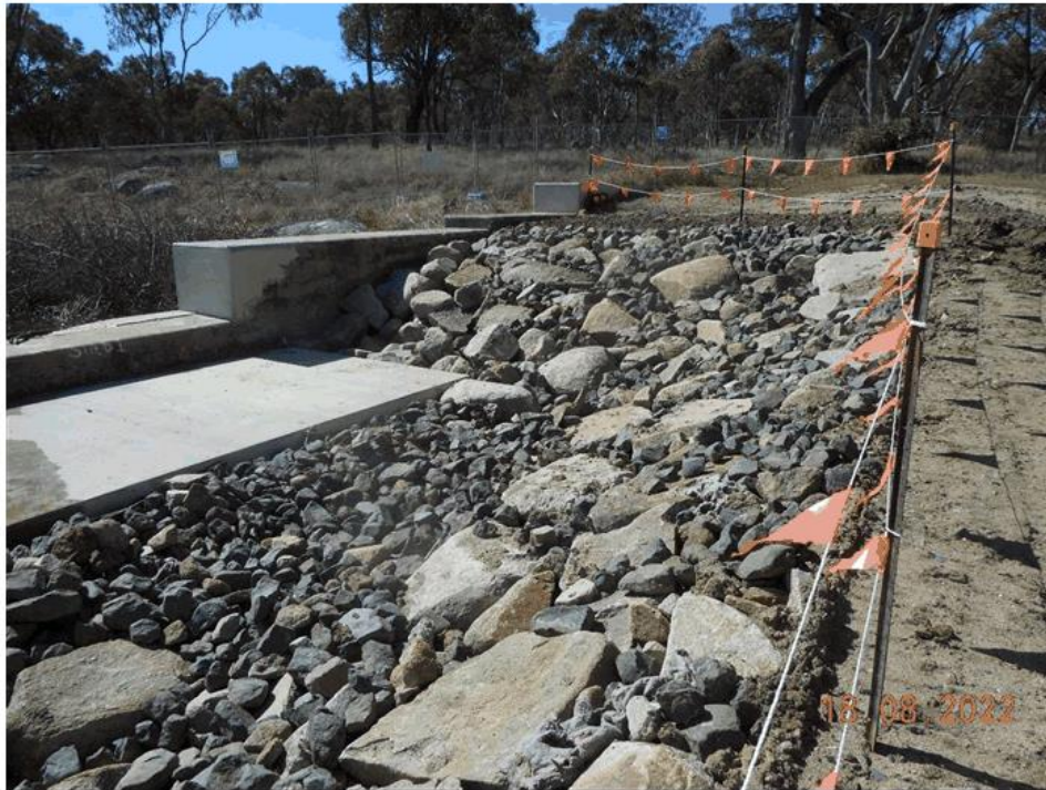
Photo Showing completed upper LH Erosion Control Slabs and Drain
