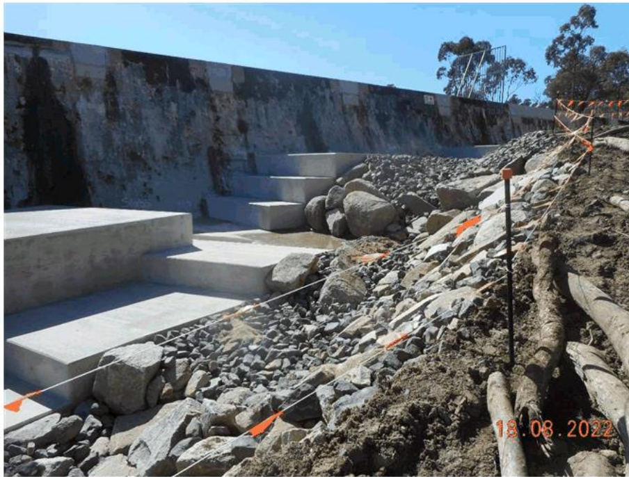
Photo Showing Stepped Section Above the Boulder
