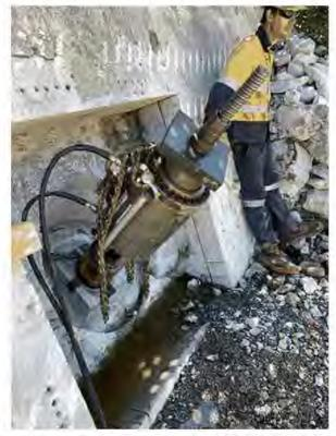
Photo Showing Stressing Jack Installed on Toe Anchor
