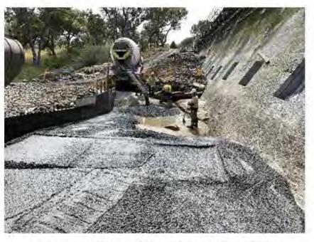
Photo Showing Toe Apron Slab Dental Concrete Installation
