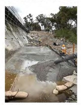
Photo Showing Toe Erosion Protection Slab Dental Concrete Pour Area
