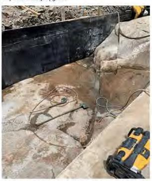
Photo Showing Toe Apron Slab Dental Concrete Preparation
