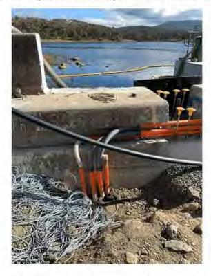
Photo Showing Monitoring Conduit Installation
