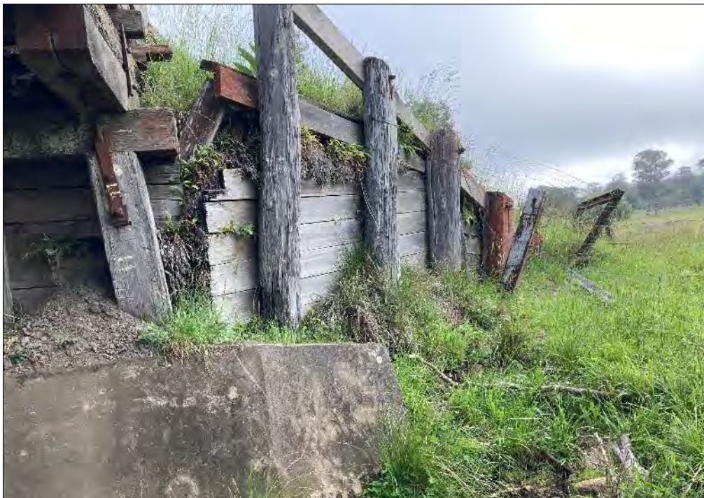
Figure 6-4: View of the typical abutment wingwall configuration and condition. The timber breastwall and wingwall planks have undergone significant deterioration and are now leaning 'outwards'. There is a loss of fines and larger aggregate from the approach through the breastwall.
