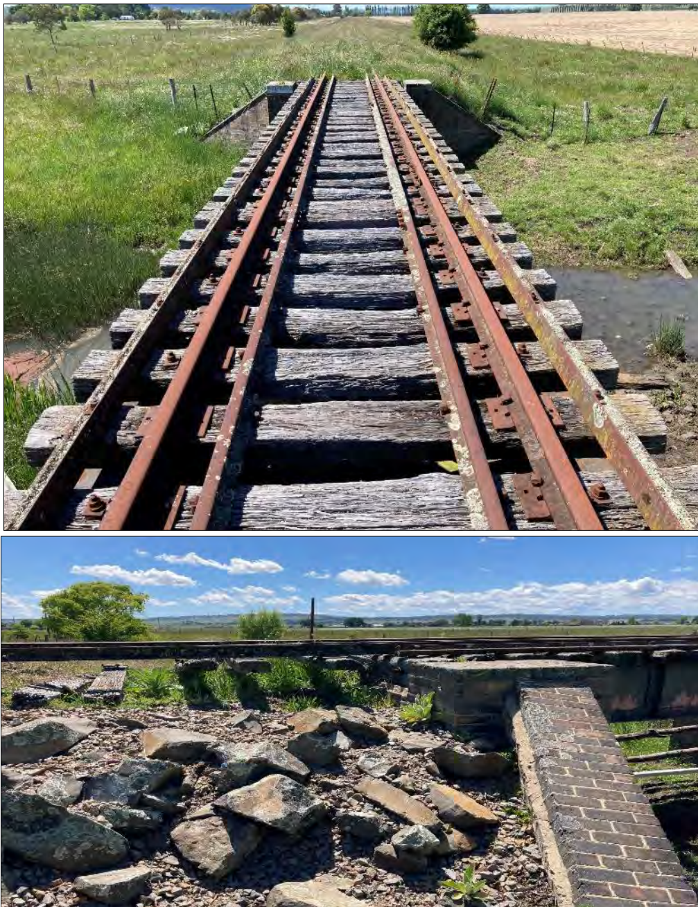
Figure 9-2: The top image is a view of the bridge looking back towards Armidale. The timber transoms are connected directly to the steel plated girders. There has been erosion/scour at Abutment 2 with many of the transoms missing and large amounts of approach fill missing. Notice the inner guard rail is still intact!!
