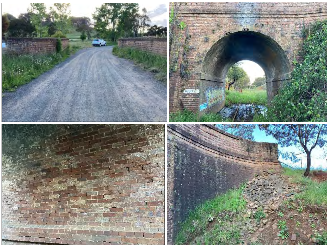
Figure 10-1: View of Crotty Road brick arch overpass bridge. This bridge is located just off the New England Highway and can be a major attraction to the trail given its historic features. The archway under the bridge is in fair to poor condition and with minor maintenance can be restored to accommodate pedestrians walking through.
