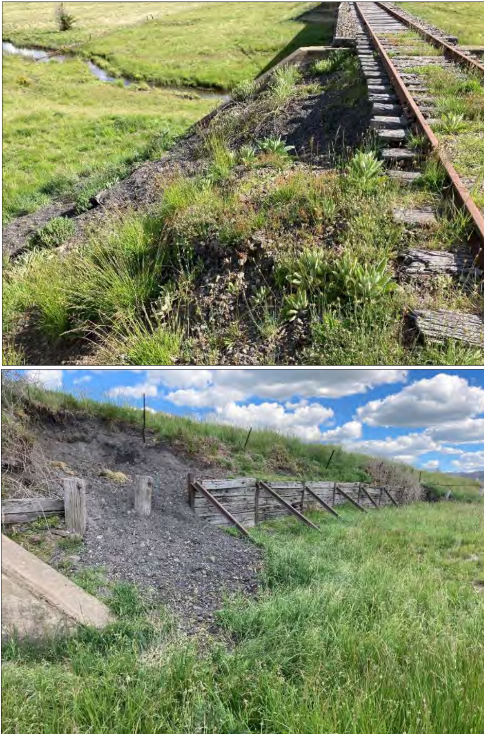
Figure 5-7: View of the typical approach configuration. The formation of the line has been significantly raised to pass over the creek which has resulted in steep unstable slopes on each side/end. The approach retaining wall is in very poor condition and requires repair to achieve a safe and stable approach formation.
