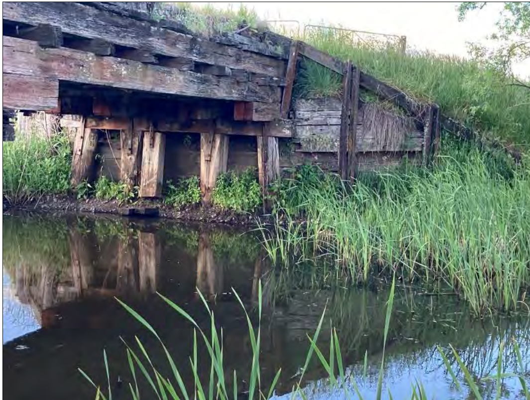
Figure 7-4: View of the typical abutment wingwall configuration and condition. The timber breastwall and wingwall planks have undergone significant deterioration and are now leaning ‘outwards’. There is a loss of fines and larger aggregate from the approach through the breastwall. Also note the very poor condition of the Abutment 2 piles where the central pile is ‘suspended’.
