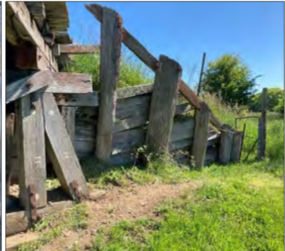
Figure 8-9: View of the typical abutment wingwall configuration and condition. The timber breastwall and wingwall planks have undergone significant deterioration and are now leaning ‘outwards’. There is a loss of fines and larger aggregate from the approach through the breastwall. The top image is Abutment 1 with the bottom image Abutment 2.
