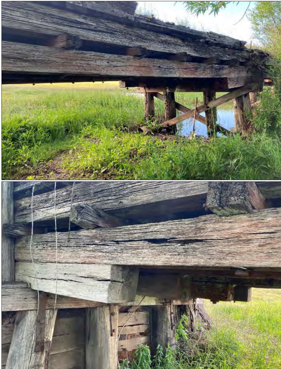
Figure 7-2: The superstructure and deck are the same configuration and similar condition as Manrowan Creek Bridge. The girders are in very poor condition with Girder 4 in Span 1 having visible cavities and excessively deflecting under its own deadload which has result in full length cracking.
