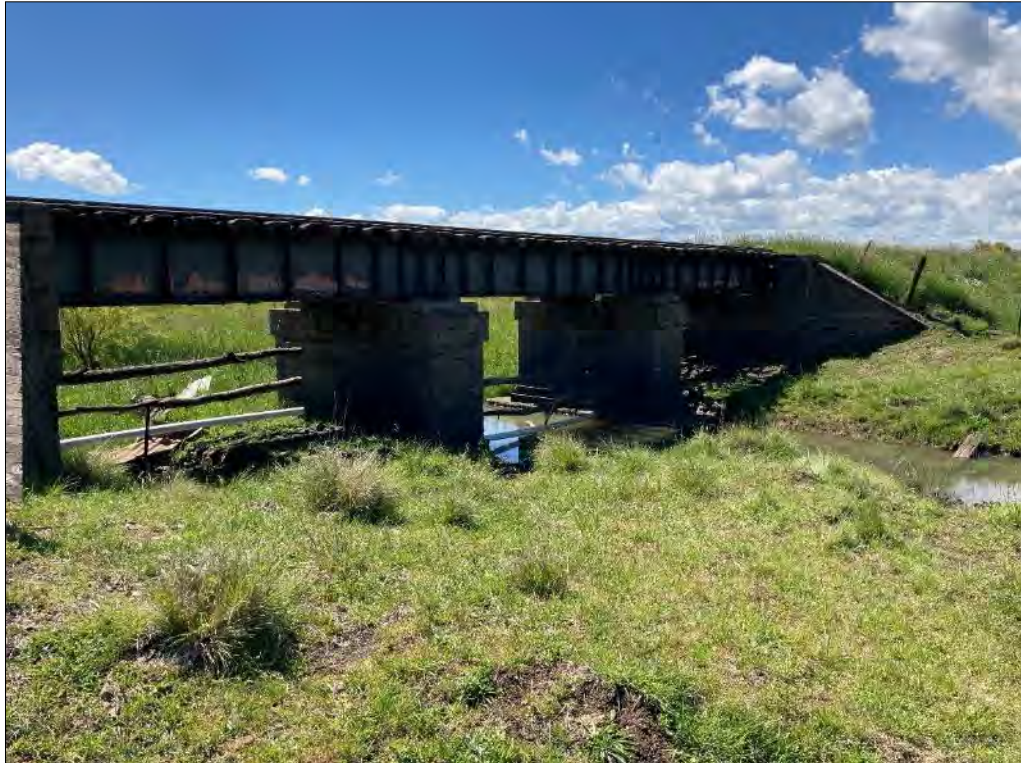
Figure 9-1: View of Stonehenge Creek Bridge from Abutment 2 end of the bridge. Abutment 1 (Southern end) is to the right side of the image above. The natural flow of the creek is through span 2 with no water flow at the time of inspection. The configuration and current condition of the bridge is similar to Upper Williams Creek Bridge with the brick pier(s) however the girders are steel plated which is very common for railway bridges. The steel girder bridge is only 3 spans long and approximately 18 metres in length. The bridge piers can be saved for aesthetics.
