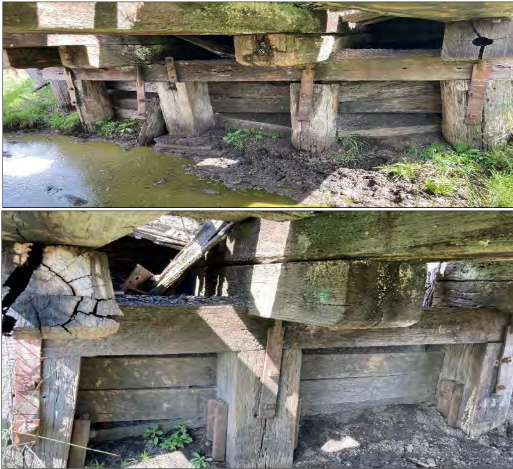
Figure 4-4: More evidence of decay present as there is large fungi growth on most elements. Brief NDT testing was completed using non-destructive methods, such as EPHOD® Stress Wave Technology. Refer to Appendix A for more information of this type of testing method. Readings above 2000-3000 \mu s was recorded for the time taken for the compression wave to travel across the section of the member tested. This was recorded on most elements. Deterioration of this magnitude means that the Modulus of Elasticity/Modulus of Rupture in various stress directions (wood is anisotropic with different strength properties in different directions) has deteriorated to an extent that the element can no longer support its own dead weight. Readings between 1000 \mu s and 2200 \mu s indicate that the member cannot carry its own dead weight in these regions. Readings in excess of 2200 \mu s can signify a cavity while a reading above 3300 \mu s indicates the element can no longer support its own dead load and is at risk of failing at any point. Refer to Section 4.3 below for a full list of recommended repair options for refurbishment to a pedestrian/cycle bridge.
