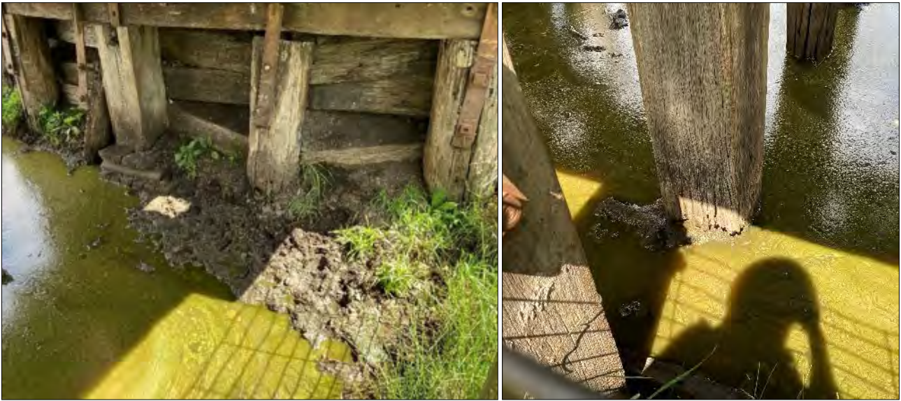
Figure 4-2: View of the timber abutments and pile. The bents comprise of 4 piles with significant deteriorated found and evident with timber packers placed under some piles (Pile 3 in the left-hand image above). Overall the timber bents were found to be in very poor condition with a complete re-build required. Breast walls were burst and pile to cap connection was lost.
