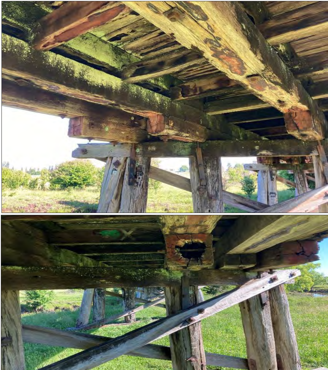
Figure 8-4: A view of the underneath section of the bridge. The superstructure comprises of 4 girder lines per span with the 2 girders per a girder line (8 girders per span in total). The double stacked square cut solid sawn girders are separated by traverse beams that contribute to the load sharing ability of the superstructure. Generally the transverse beams were in poor condition and the girders are in poor-very poor condition. One of the girders has undergone significant deterioration with large splits visible from the underneath as well as being covered fully in decay fungi growth. The girders and corbels are connected with large vertical through bolts. Vertical fasteners increase the rate of decay in timber as they allow moisture to travel down the fastener into the heartwood of the girders and corbels where evaporation is more difficult, therefore increasing the moisture content in the middle of these elements over longer periods of time. The heartwood of a large dimensional element is less capable of breathing and expelling moisture than the sapwood that surrounds it, so vertical connectors funnel the moisture directly into the heartwood accelerating decay. Once the moisture content exceeds 22%, timber consuming fungi are activated and the decay process begins. Refer to Figure 3-2 for a detailed description of how and where the decay occurs due to these vertical bolts.
