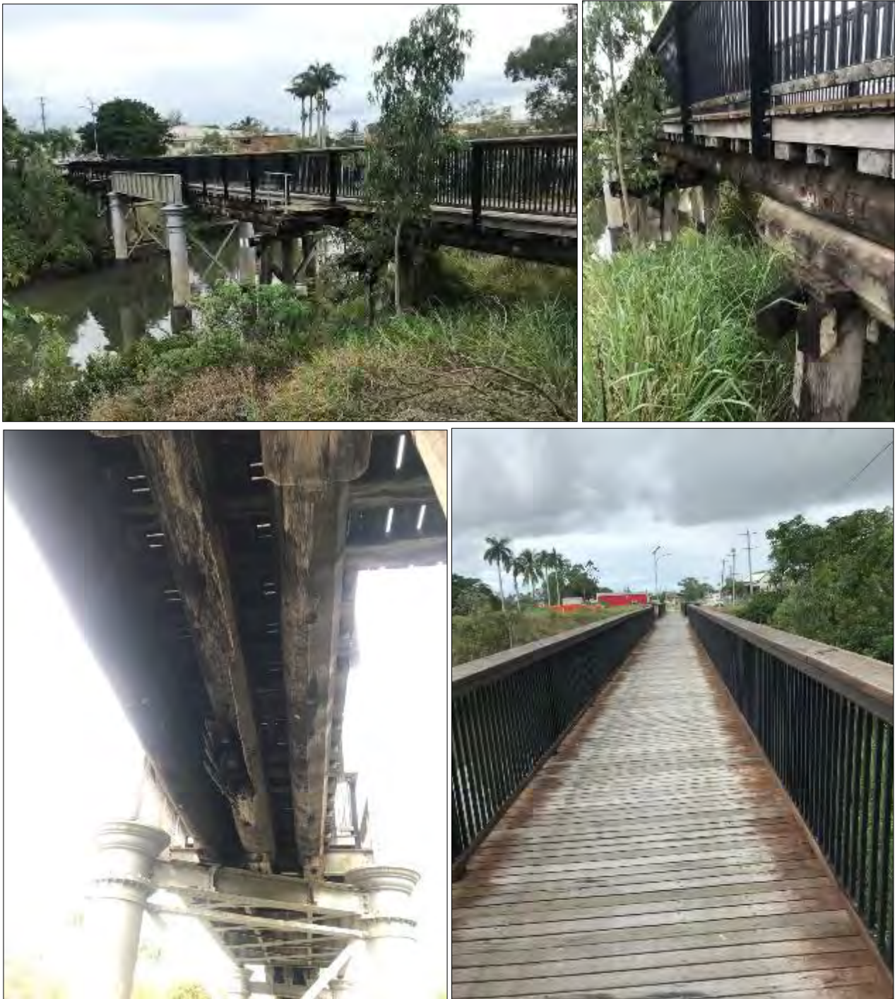
Figure 11-2: The above photo series demonstrates a similar repair to the option explored but deemed not viable for this rail trail. The existing railway bridge was left un-touched and a new hardwood deck system with handrails was installed. Six 100mm x 250mm timber joists were placed on top of the existing transoms (rail ties) with a 38-50mm thick hardwood deck installed on top. This option will likely be the lowest cost but also carries the shortest expected lifespan. As seen in the bottom left photo above, one of the girders has failed and fallen out creating a ‘weak’ point along the bridge. Due to a high residual capacity of timber and the continuous joists, a complete failure of the bridge (span) hasn’t occurred yet but is only a matter of time unless extensive maintenance is undertaken.
