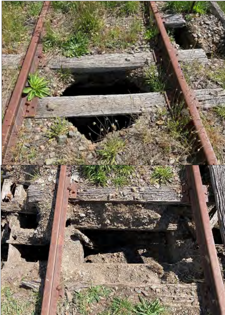
Figure 4-5: The timber transoms (rail ties) were found to be in a poor condition with fouled ballast and lost ballast. If the bridge was to be repurposed for pedestrian and cycle use the timber transoms, railway line and rock ballast would be required to be removed. The existing timber edge rail that contains the ballast can left in place to act as a kerb/kick rail in the repurposed bridge. To meet the current standards and Australian codes; vertical balustrade panels and a 1.4m high cycle rail will need to be installed. The current width of the bridge from inside of kerb to inside of kerb is approximately 3.0 metres which will result in a code compliant width for pedestrian bridges. As many of the deck planks are ‘falling’ out a new deck would be required for this bridge.
