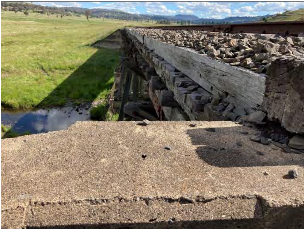
Figure 5-9: View of Side 2 (Right-hand side) of the bridge from Abutment 2. The bridge maintains a fairly straight alignment while the decay of the bents/girders are visible to the uneven ‘drops’ along the length of the bridge. The ballast tray remains intact with most of the ballast.
