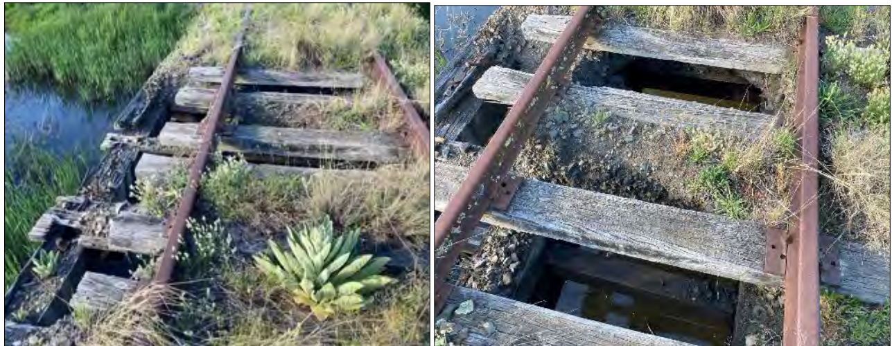
Figure 7-5: The deck planks that support the ballast rock are in very poor condition with many of the planks missing and large amounts of ballast have fallen out. To meet the current standards and Australian codes; vertical balustrade panels and a 1.4m high cycle rail will need to be installed along with a new deck system.
