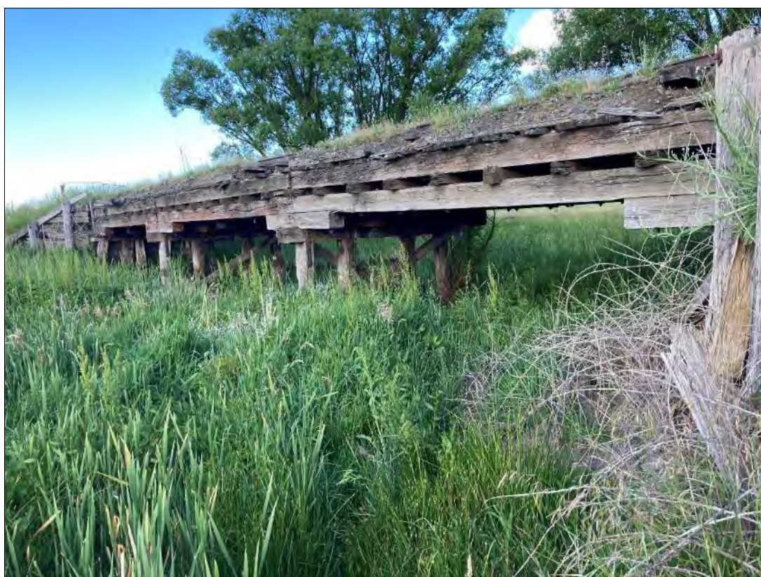
Figure 7-1: View of Williams Creek from Abutment 1 end of the structure. The 3 span, 24m long bridge has the same superstructure and deck configuration as Manrowan Creek Bridge with timber pile bents. There is a large amount of vegetation growth around the bridge which keeps the moisture content high in the timber. When the moisture level in the timber is above 22%, decay-causing fungi can start to grow; when the moisture content drops below this level, the fungi become dormant and decay will be arrested until the moisture content rises again.
