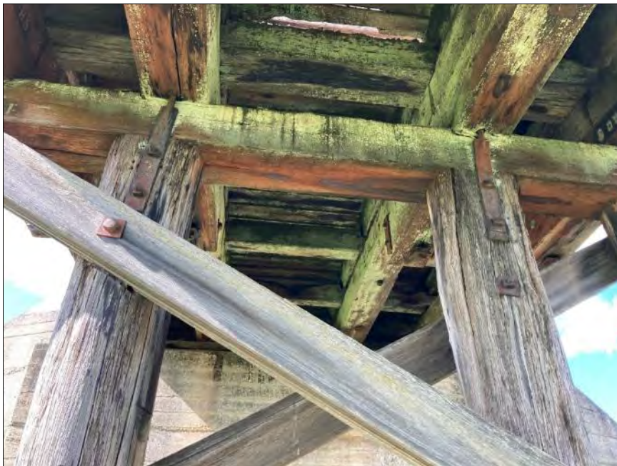
Figure 5-6: Close-up view of the approach span. The members are connected with a vertical through bolt. Vertical fasteners increase the rate of decay in timber as they allow moisture to travel down the fastener into the heartwood of the girders and corbels where evaporation is more difficult, therefore increasing the moisture content in the middle of these elements over longer periods of time. The heartwood of a large dimensional element is less capable of breathing and expelling moisture than the sapwood that surrounds it, so vertical connectors funnel the moisture directly into the heartwood accelerating decay. Once the moisture content exceeds 22%, timber consuming fungi are activated and the decay process begins.
