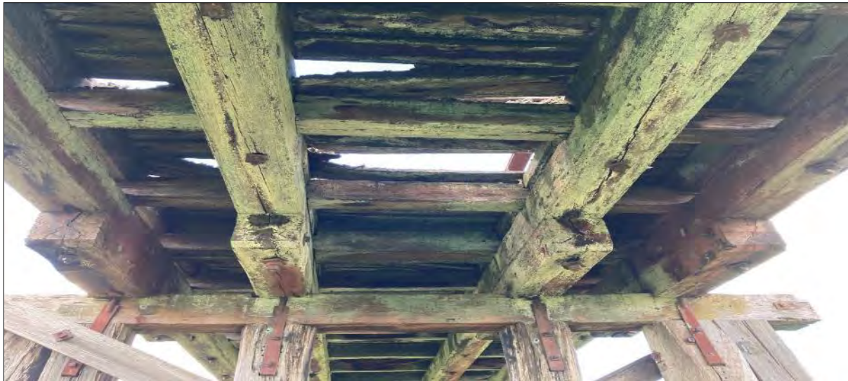
Figure 5-5: A view of a section of the deck that has collapsed. These planks will require replacement before the bridge can be reopened for pedestrian and cycle use. The ballast rock will also be required to be removed to accommodate pedestrian and cycle traffic. Large amounts of decay fungi growth evident which indicates large amount of deterioration present.
