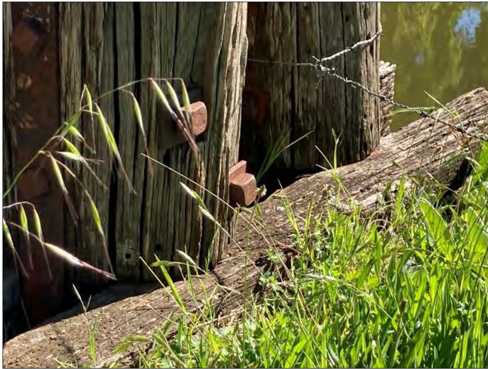
Figure 8-3: It was noted that the bottom section of several posts and timber cap wales have started to undergo decay. This is as expected due to the timber posts bearing directly on the concrete footing which typically has a high moisture content. Over time the timber post undergoes capillary action and draws up the moisture like a ‘straw’. Once the moisture content in the timber elements reaches 22%, decay causing fungi are activated and the decay process begins. Overall the timber bents were found to be in poor condition. The bottom sections of the timber piles were determined to be a ‘hotspot’ for decay and determined to be an ideal area to test using non-destructive methods, such as EPHOD® Stress Wave Technology. Refer to Appendix B for more information of this type of testing method. A reading of above 1500µs was recorded for the time taken for the compression wave to travel across the section of the member tested. This was recorded at the bottom of one of the piles (left image above) and was found to be similar across most of the piles/posts. Deterioration of this magnitude means that the Modulus of Elasticity/Modulus of Rupture in various stress directions (wood is anisotropic with different strength properties in different directions) has deteriorated to an extent that the element can no longer support its own dead weight. Readings between 1000µs and 2200µs indicate that the member cannot carry its own dead weight in these regions. Readings in excess of 2200µs can signify a cavity while a reading above 3300µs indicates the element can no longer support its own dead load and is at risk of failing at any point.
