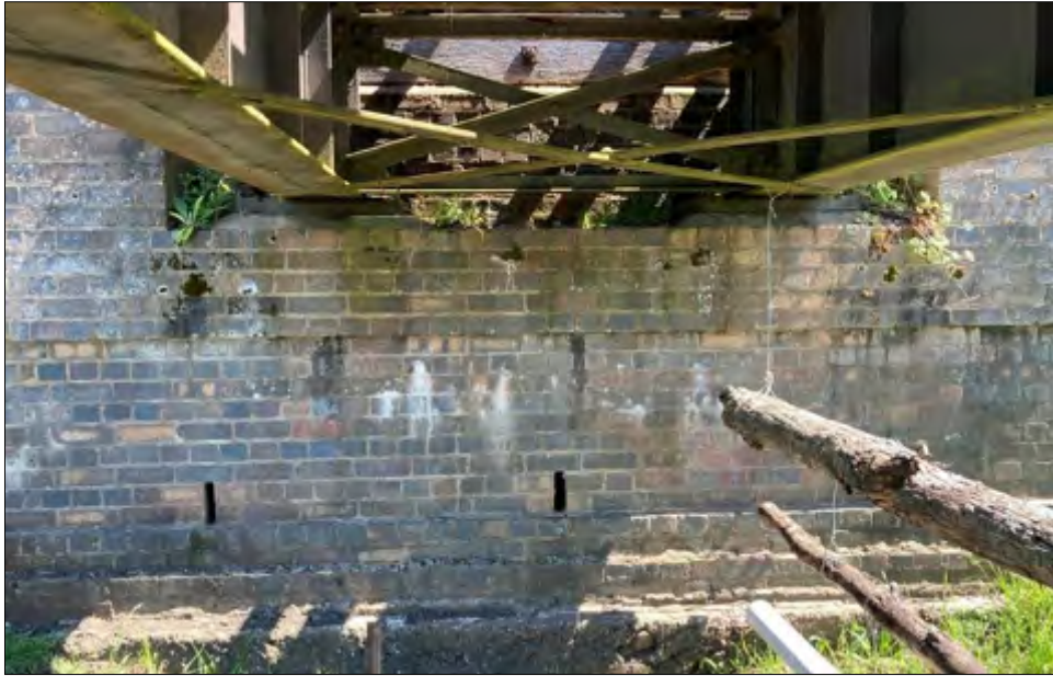
Figure 9-3: View of the brick Abutment that is approximately 3 metres in height. The steel plated girders bear directly on the brick pier. The girders are lateral supported by transverse and diagonal bracing. The substructure can be preserved.
