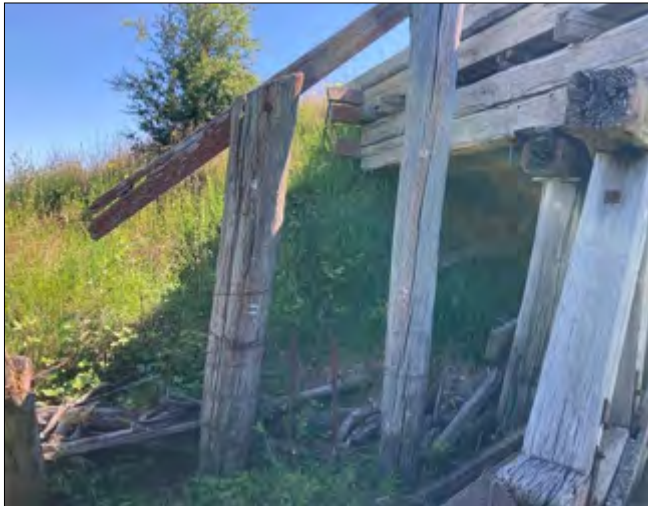
Figure 8-9: View of the typical abutment wingwall configuration and condition. The timber breastwall and wingwall planks have undergone significant deterioration and are now leaning ‘outwards’. There is a loss of fines and larger aggregate from the approach through the breastwall. The top image is Abutment 1 with the bottom image Abutment 2.
