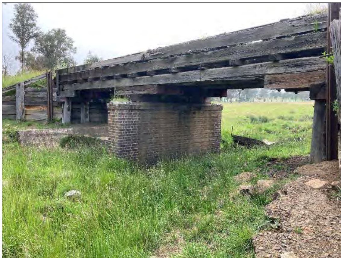
Figure 6-1: View of Upper Williams Creek Bridge from Abutment 1 end of the bridge. Abutment 1 (Southern end) is to the right side of the image above. The natural flow of the creek is through span 2 with no water flow at the time of inspection. The configuration and current condition of the bridge is similar to Manrowan Creek Bridge with a beautiful brick pier (which can be saved to protect the construction of the era) instead of timber bents. The timber bridge is only 2 spans long and approximately 14 metres in length.
