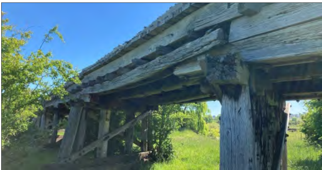
Figure 8-8: Another view of a section of the bridge that has collapsed/sunken due to the girder and corbel 'crushing' due to significant decay. The girders and corbels are connected down to the cap with a vertical through bolt. Vertical fasteners increase the rate of decay in timber as they allow moisture to travel down the fastener into the heartwood of the girders and corbels where evaporation is more difficult, therefore increasing the moisture content in the middle of these elements over longer periods of time. The heartwood of a large dimensional element is less capable of breathing and expelling moisture than the sapwood that surrounds it, so vertical connectors funnel the moisture directly into the heartwood accelerating decay. Once the moisture content exceeds 22%, timber consuming fungi are activated and the decay process begins. Refer to Figure 3-2 for a detailed description of how and where the decay occurs due to these vertical bolts.
