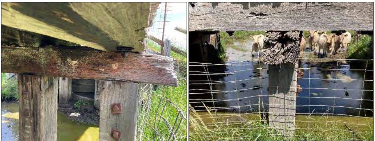
Figure 4-3: Most elements have started to undergo significant decay with Bent 1 cap visibly decayed above. Large amounts of fungi growth (white spots) are evident on most elements and is seen in the left-hand image above. Once the moisture content in the timber elements reaches 22%, decay causing fungi are activated and the decay process begins.
