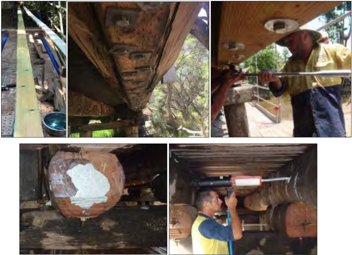
Figure 11-5: The repair of Meachams Bridge in Cassowary Coast. The bridge was retrofitted with fibre reinforcement on the bottom of the girders, some corbels and girders were injected with a high strength epoxy. Some piles were also wrapped with high strength fibre and injected with epoxy, then the entire bridge was diffused with borate salt rods to neutralize decay growth.
