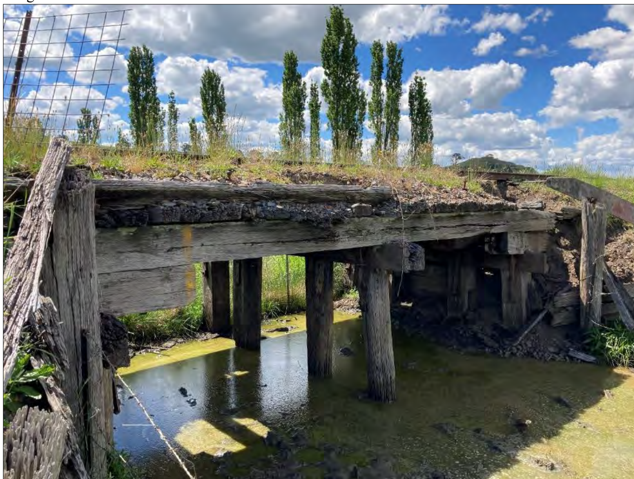
Figure 4-1: View of Old Ben Lomond Rd Bridge from Abutment 1. The timber bridge is 2 spans long and approximately 8 metres long. At the time of inspection, the water was not flowing (boggy ‘spring’) and had a maximum depth of 0.5m. The wingwalls and backwalls have significantly deteriorated and no longer retain any of the approach fill material. Also note there is a fence located/attached on the left side of the bridge. Also note the horizontal crack on Girder 4 which is a key sign of internal decay and section loss causing the beam to fail under the deadweight of the bridge alone.
