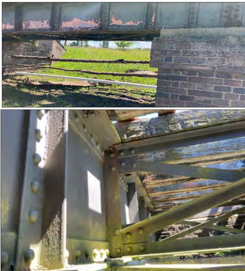
Figure 9-4: The steel is starting to show signs of corrosion with maintenance required for the steel plated beams. A lightweight deck system on-top of the girders will be the recommended repair solution for this bridge combined with steel repairs.
