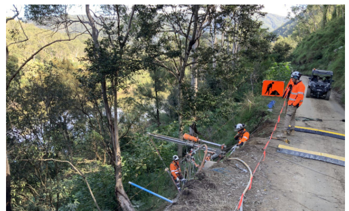
Soil nail works at Flying Fox Cutting
