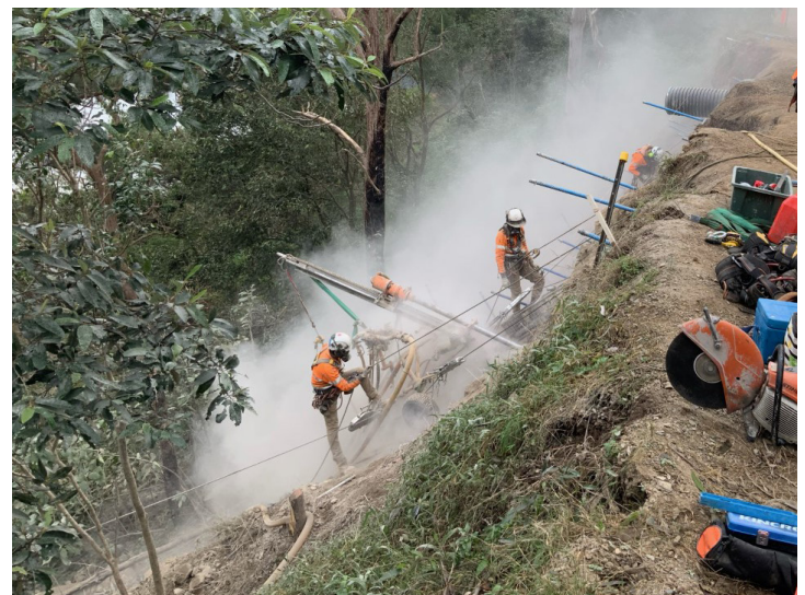
Soil nailing works underway
