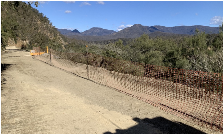
Road widening works at Flying Fox Cutting
