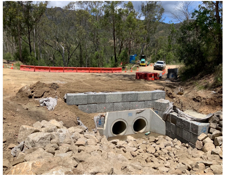
Curve 3 culvert works
