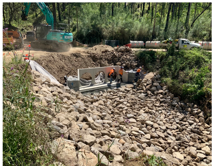
Curve 2 culvert works
