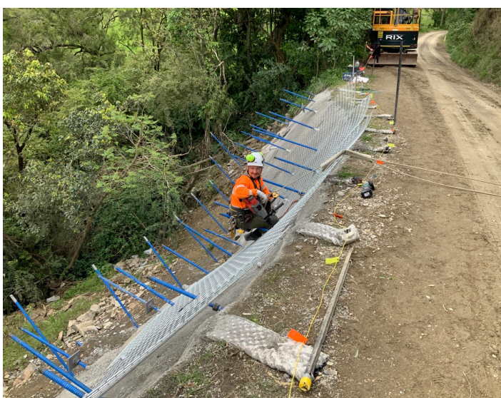
Smith's Bluff soil nail stabilisation works
