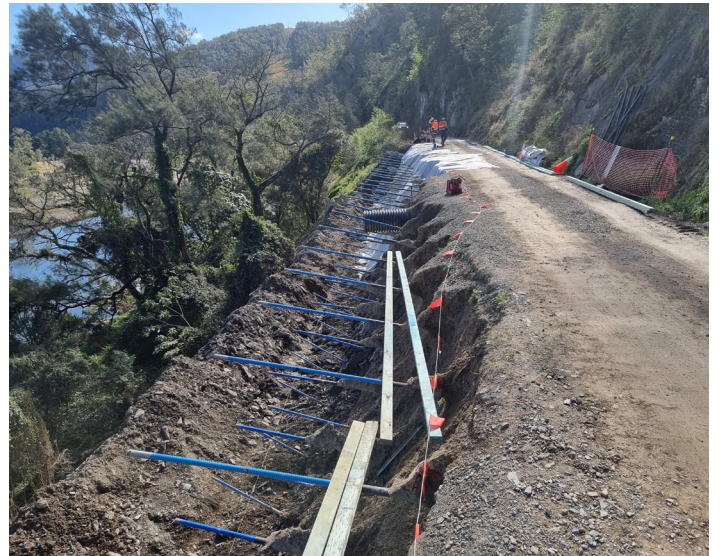
Flying Fox Cutting soil nail stabilisation works
