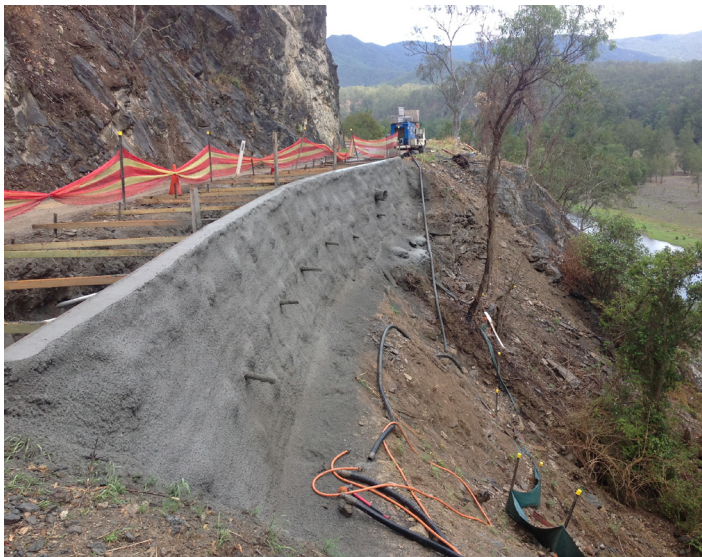
Flying Fox Cutting shotcrete in place
