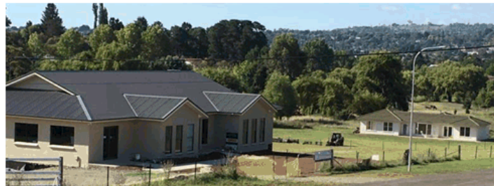
(Looking south-east): Foreground – Lot 2 containing health consulting rooms, background – Lot 3 containing relocated dwelling.
