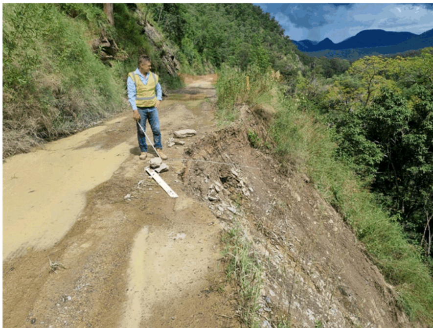
Figure 3 AGRN 1012 – Hillside stripping and moderate landslide in narrow roadway, area currently under emergency repair
