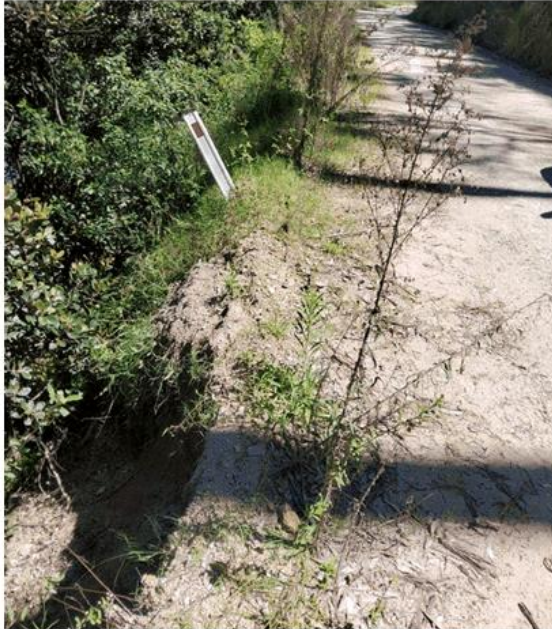
Figure 2 AGRN 1012 Damage – Loss of hinge and propagating damage
