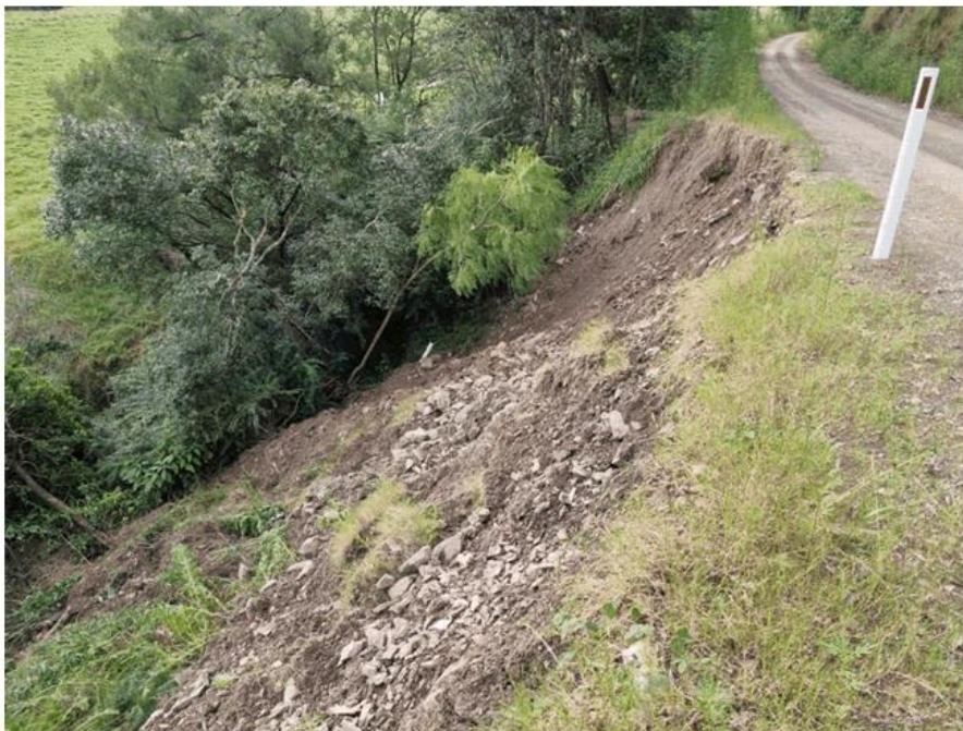
Figure 2 AGRN 1012 Damage – Loss of hinge and propagating damage
